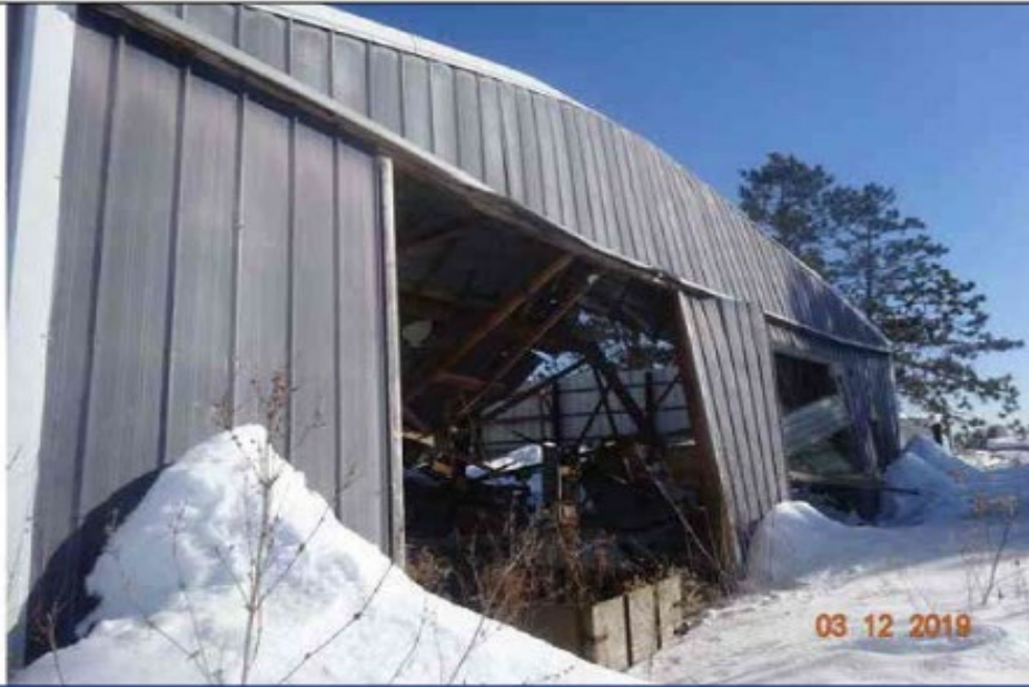
Photo 21: Displaced south wall.
