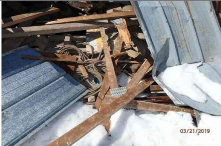
Photo 19: Fractured truss members.
