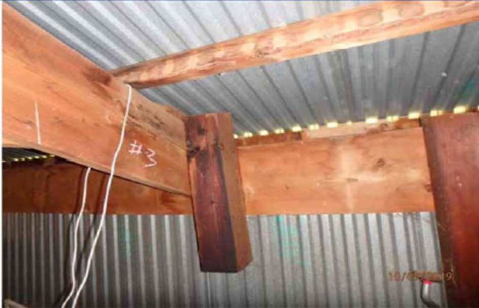
Photo 20: Truncated column and header/ledger board.
