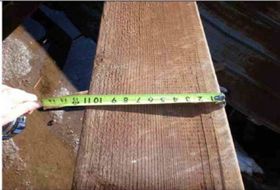
Photo 15: Top chord depth which scale.
