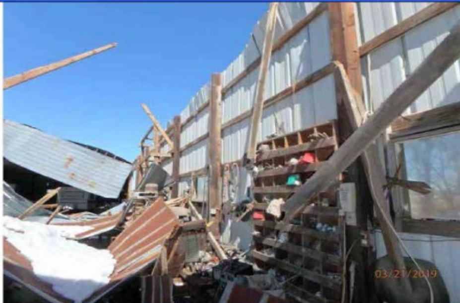
Photo 20: Displaced columns and deformed panels.
