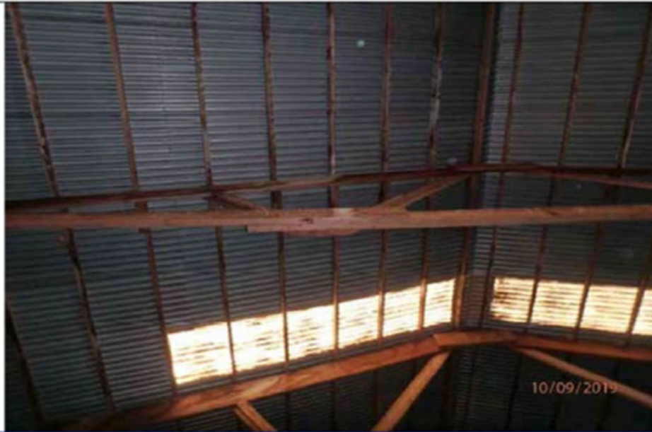
Photo 11: Typical bottom chord lap splice.
