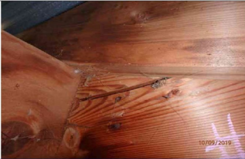
Photo 19: Alternate view of aged fracture in previous photo.
