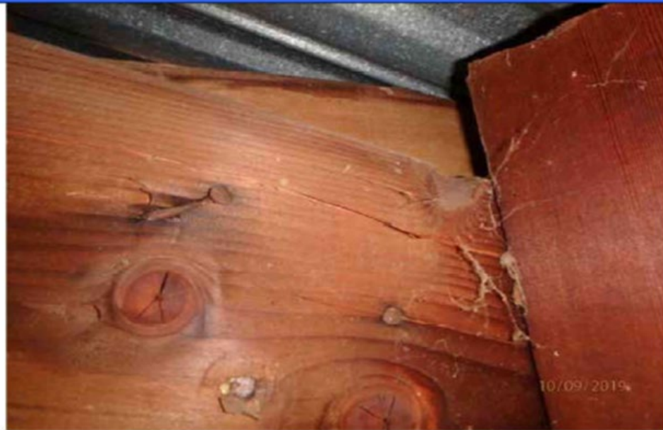
Photo 22: Alternate view of fracture in previous photo.
