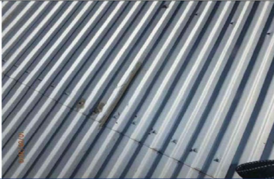
Photo 7: Sealant at panel side lap.
