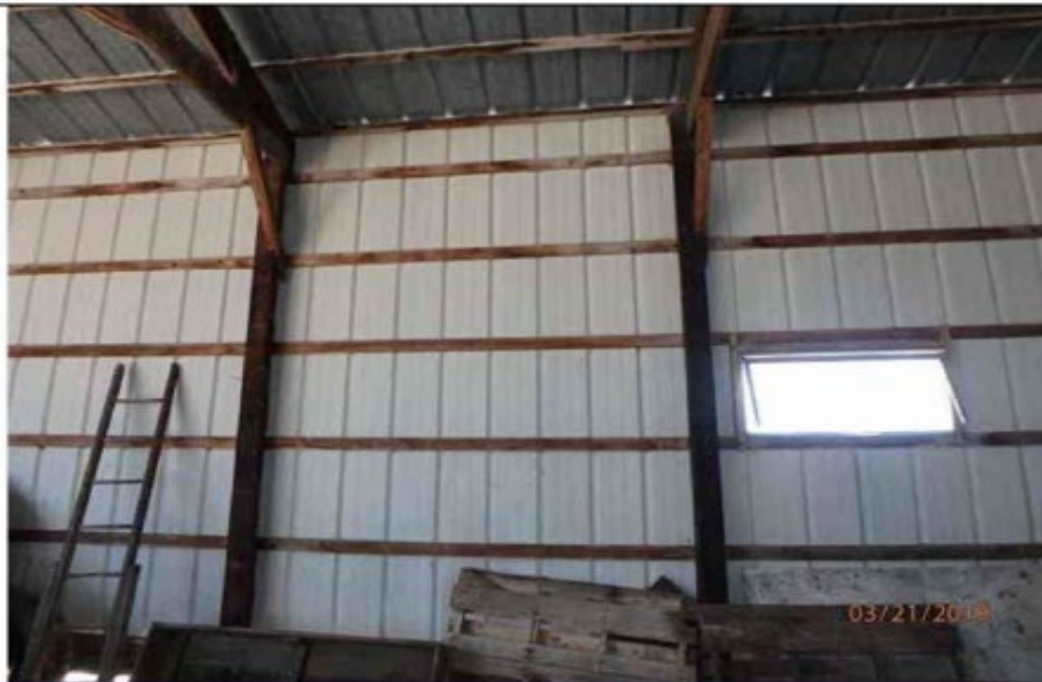
Photo 7: Typical wall framing.
