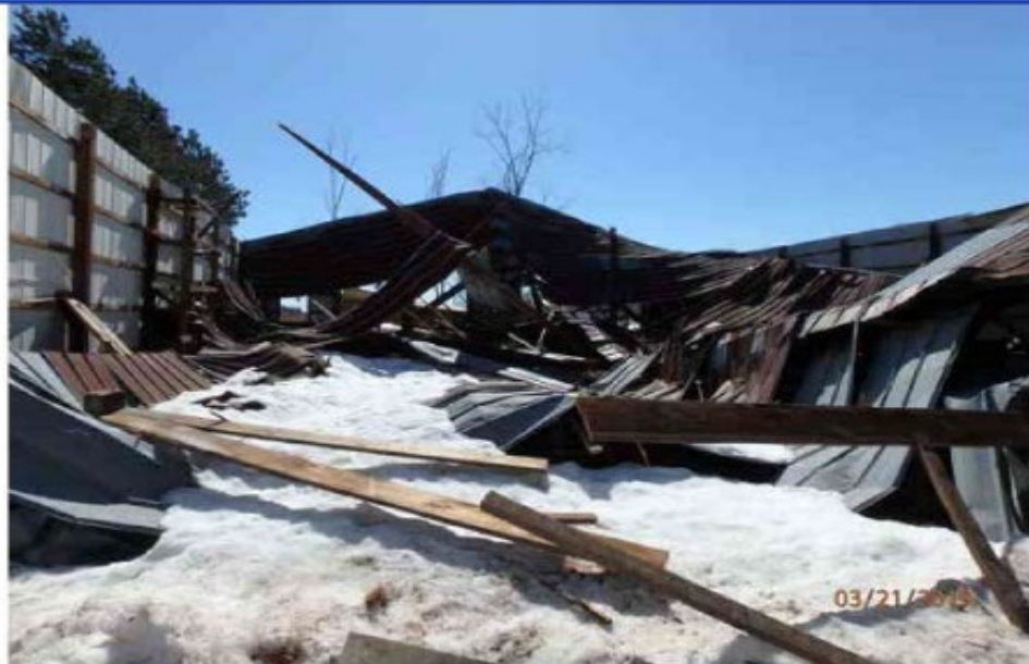
Photo 18: Snow build-up east side of building.
