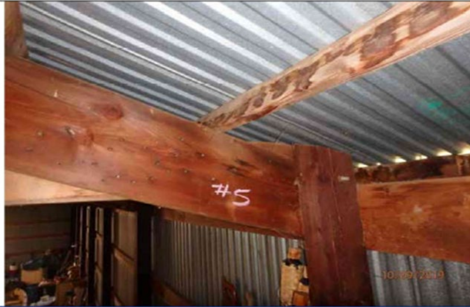
Photo 23: Horizontal shear fracture (aged appearance).
