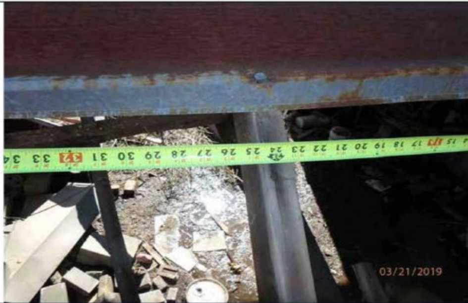
Photo 17: Purlins spaced at 24" o.c.
