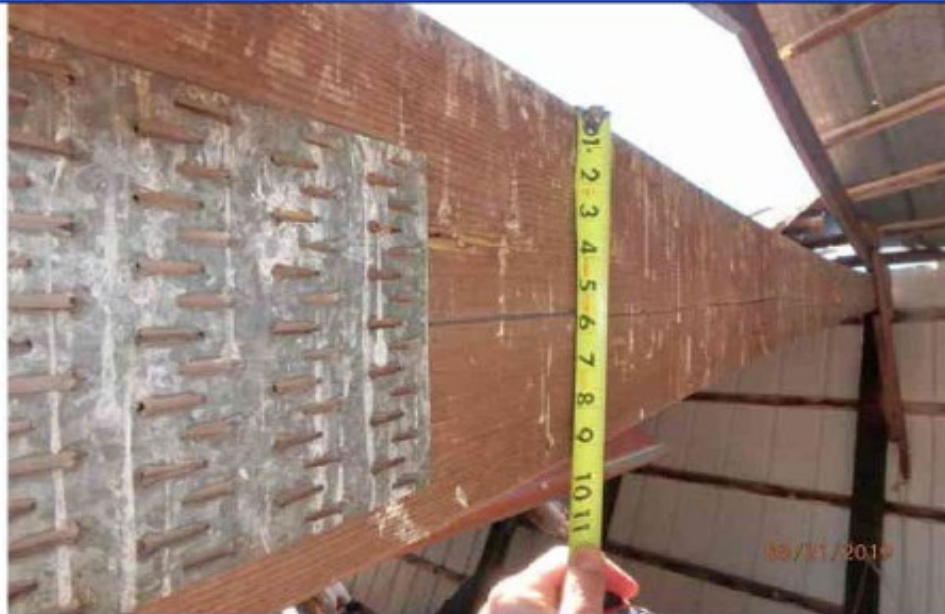
Photo 14: Bottom chord depth with scale.
