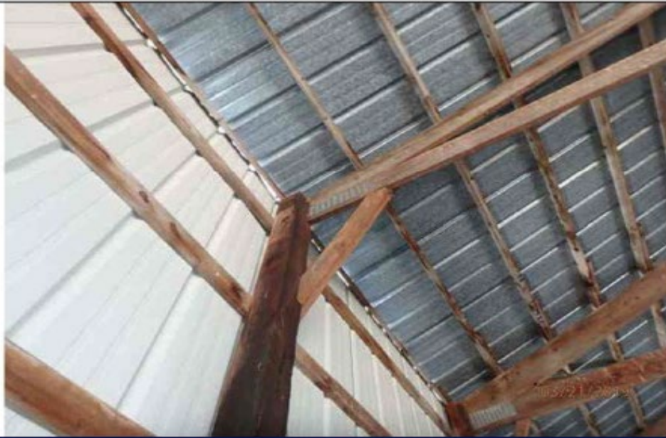
Photo 9: Typical column/truss connection.
