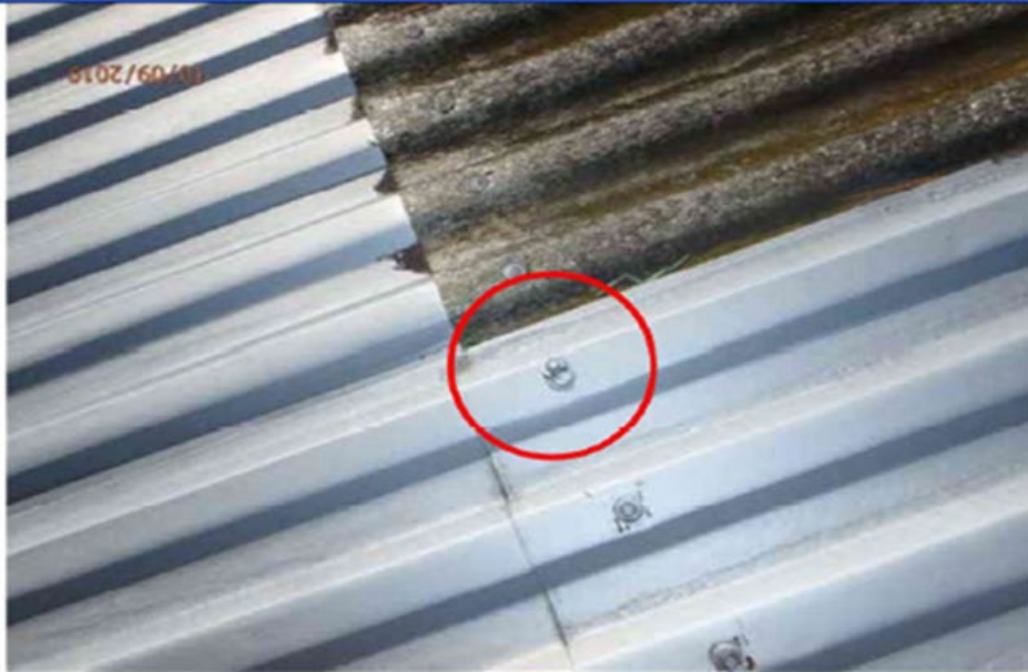
Photo 8: Multiple fasteners.
