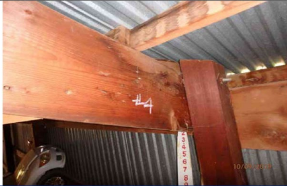
Photo 21: Horizontal shear fracture (new appearance).
