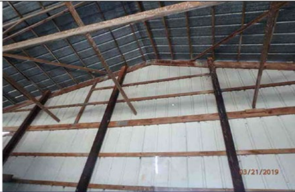
Photo 13: Detached bracing at north wall.
